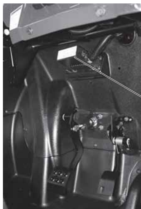
Main Fuse Box
